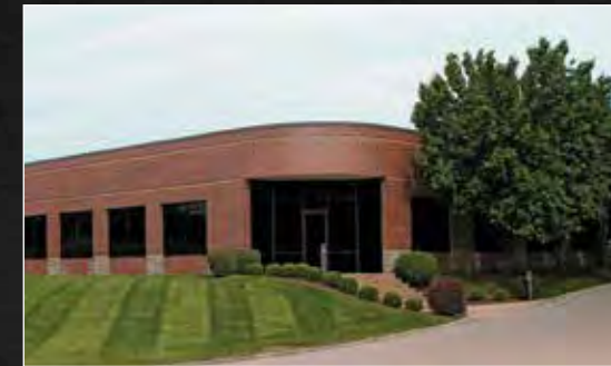
STEEL PREPARATION FACILITY St. Charles, Missouri, USA
