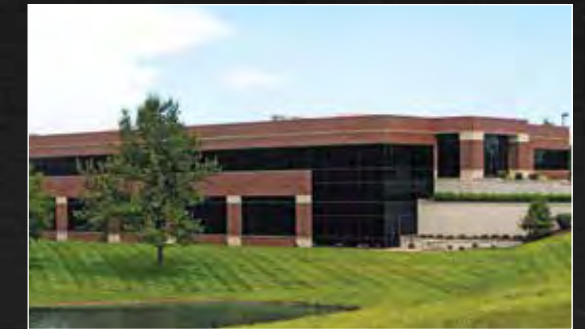
TECHNICAL TRAINING & PRESS REFURBISHING FACILITY St. Charles, Missouri, USA
